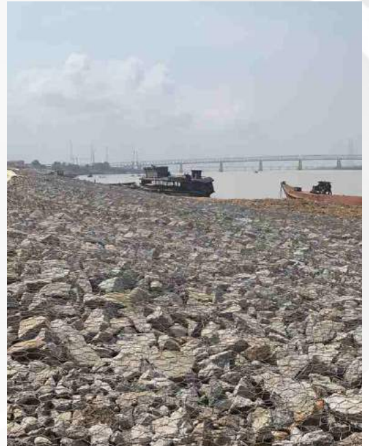
Gabion type Shore Protection works at the bank of River Niger at Ose, Ogbe-Ijaw, Onitsha, Anambra state
